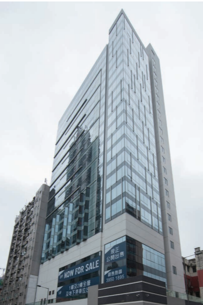
Hong Kong KHORA (Modernised industrial building)
